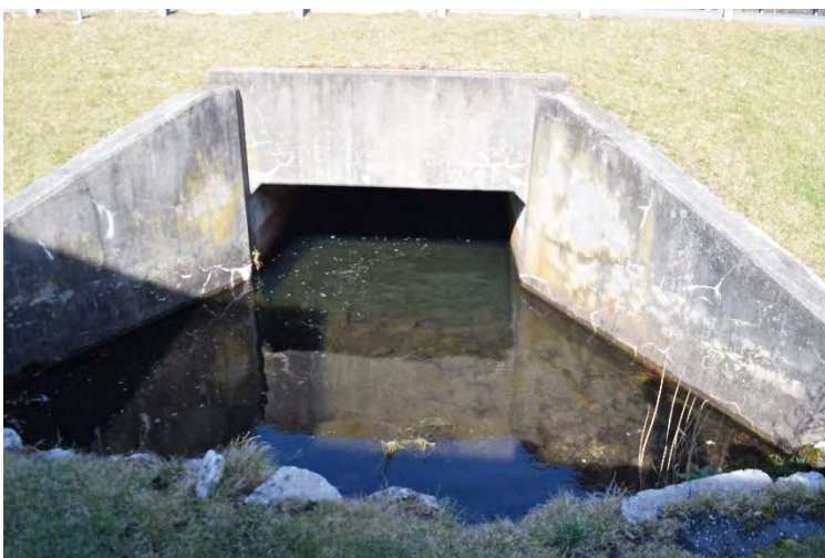
Culvert north of Mill
