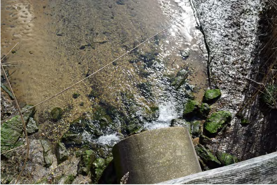
Pipe South of Old Montauk Highway
