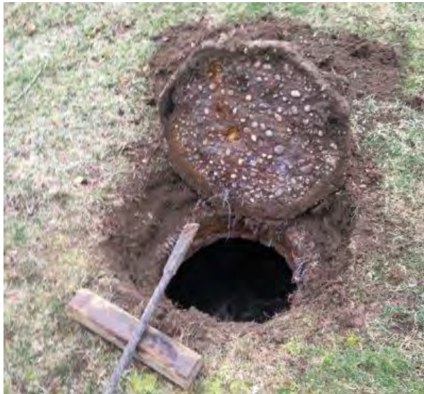
Cesspool-ineffective method of treating wastewater.
