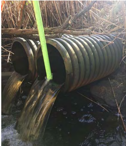
Figure 8: Downstream end of culverts at Stepping Stone Pond. Culverts perched approximately 1' above bed of channel.
