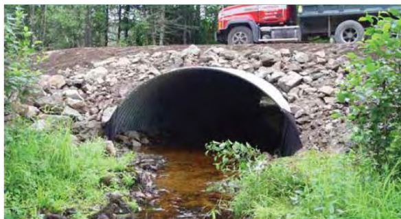
Figure 17: Pipe arch culvert, photo courtesy of Downeast Lakes Land Trust. The diagram on the right is a schematic detail of this type of culvert depicting stream bed materials placed in the bottom of the culvert.
