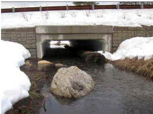
Figure 11: An example of a concrete box culvert with natural channel substrate on the bottom and a floodplain bench built for terrestrial organism passage.
