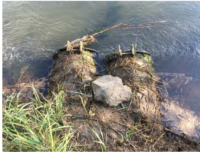
Right: Culverts with Tide Gate
