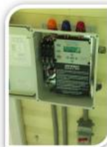
Standard I/A OWTS Control Panel
