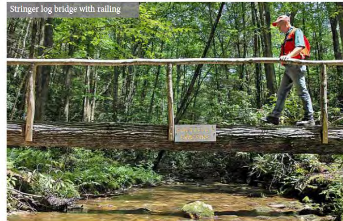
Stringer log bridge with railing
