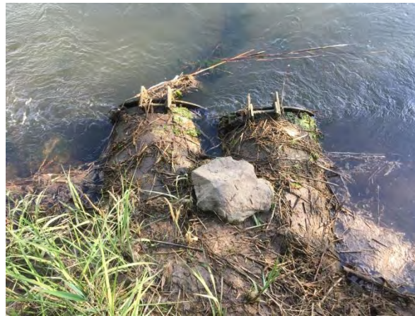
Center: Culverts with Tide Gate
