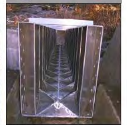
Cross-section: Alaskan Steeppass Ladder
