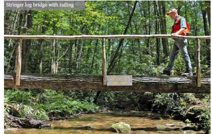
Stringer log bridge with railing
