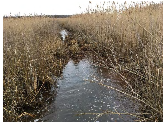
Main Ditch to Peconic River: Obstruction Looking Upstream (top) Obstruction Looking Downstream (bottom)
