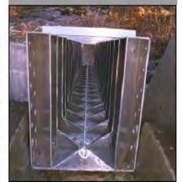
Cross-section: Alaska Steeppass Ladder
