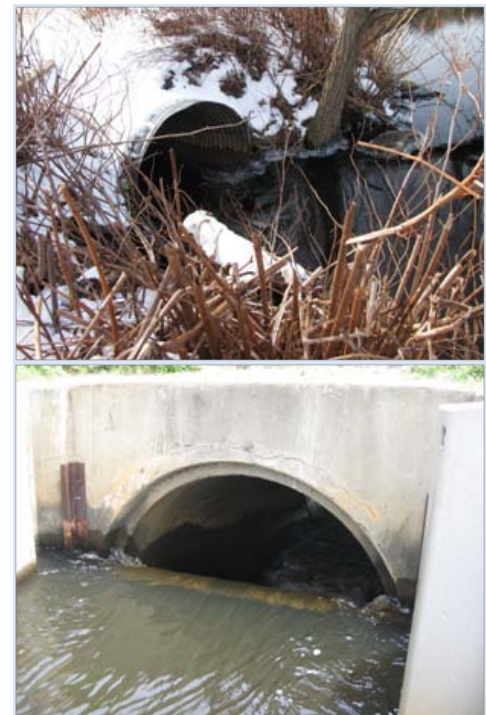
Figure 9. (Top) Looking downstream at the north culvert; (bottom) looking downstream at the south culvert with stop logs in place.
