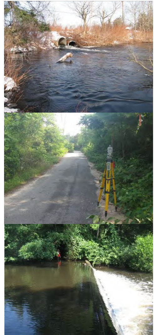
Figure 2. (Top) Looking upstream at the Upper Mills Dam and the downstream outlets of the two culverts; (middle) looking north along the paved road on top of the dam; (bottom) looking north at the USGS gaging weir downstream from the dam.
