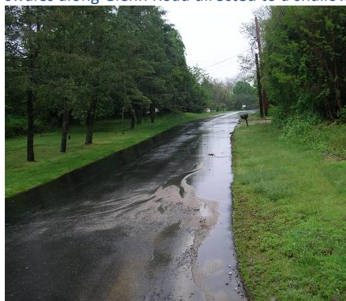
Figure 4.10. Sedimentation along Glenn Road (left). Proposed retrofit (right) would involve construction of dry swales along Glenn Road directed to a shallow bioretention area that would overflow into the existing inlet.
