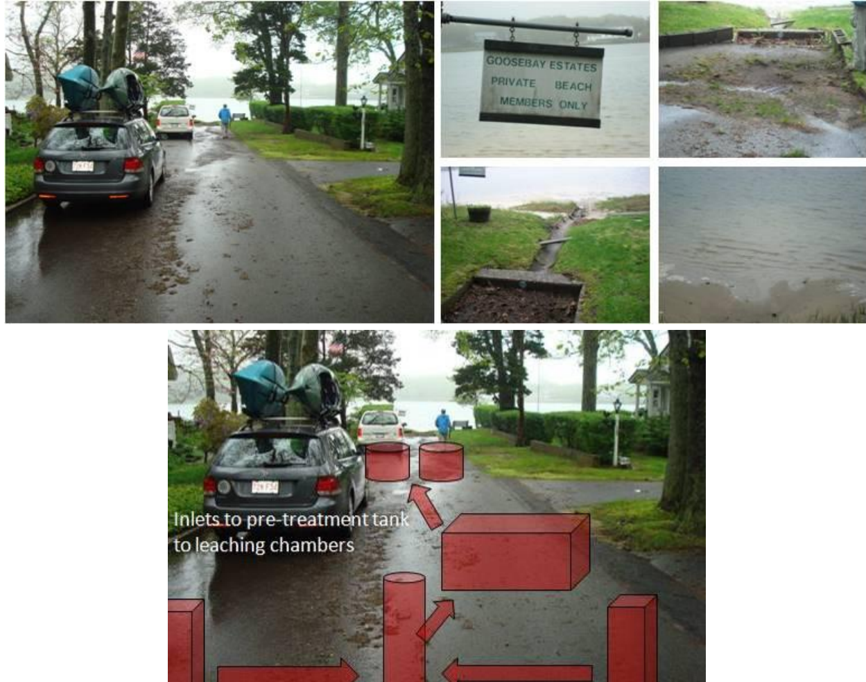
Figure 4.16. Existing conditions at the end of Pine Avenue where stormwater runoff results in an accumulation of sediments that have created a delta within Goose Creek at a private beach (top photos). Proposed stormwater retrofit concept would involve traditional structural measures to address the steep slopes and relatively narrow roadway right-of-way along Pine Avenue (bottom).
