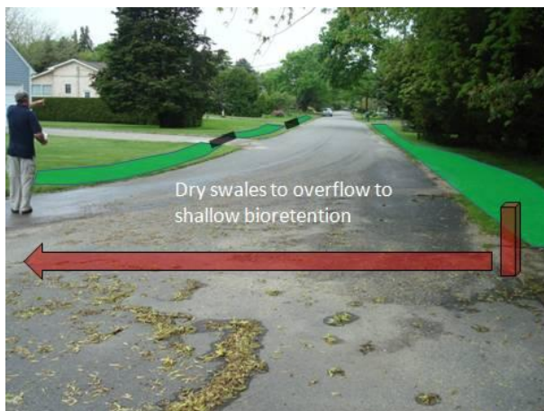
Figure 4.20. Sedimentation and ponding at the intersection with Gagens Landing Road and Clearview Avenue. Proposed stormwater retrofit would involve the installation of dry swales directed to a shallow bioretention area to allow for temporary storage and water quality treatment.
