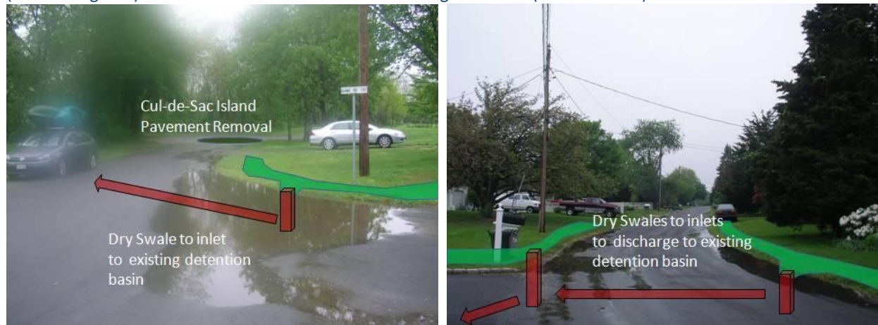
Figure 4.3. Grange Lane with views toward cul-de-sac (right) and Grange Lane Ext. (left). Proposed dry swales (shaded in green) would be directed to inlets and leaching chambers (shaded in red).
