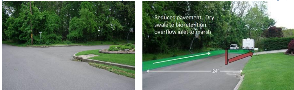
Figure 4.21. Existing conditions along Landing Path, which is located just west of a nature sanctuary (left). The proposed retrofit includes a reduction of impervious surface, a dry swale, and a bioretention area (right).
