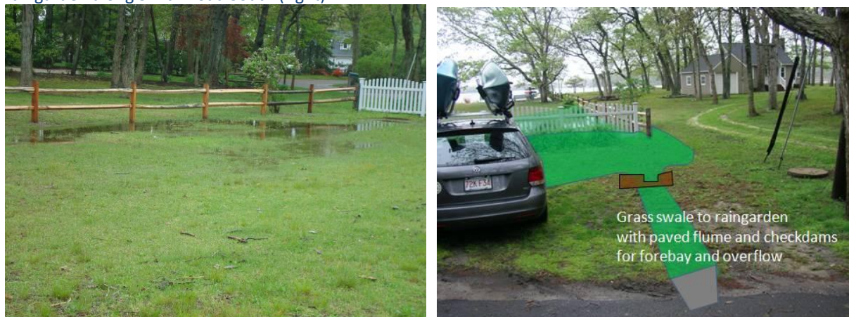
Figure 4.8. Ponding at common area (private beach) within Goose Neck Estates (left). Proposed grass swale and raingarden along Smith Road South (right).
