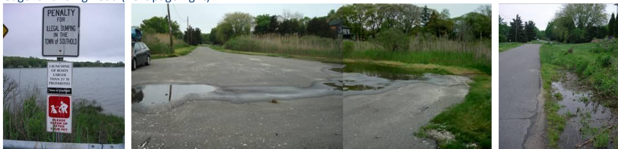
Figure 4.19. Ponding and sedimentation along Gagens Landing Road near public boat ramp (below center). The existing “wet swale” garden created by the adjacent property owner (next page left) suggests an easily implemented stormwater retrofit by extending this wet swale practice along both sides of the lower reaches of Gagens Landing Road (next page right).
