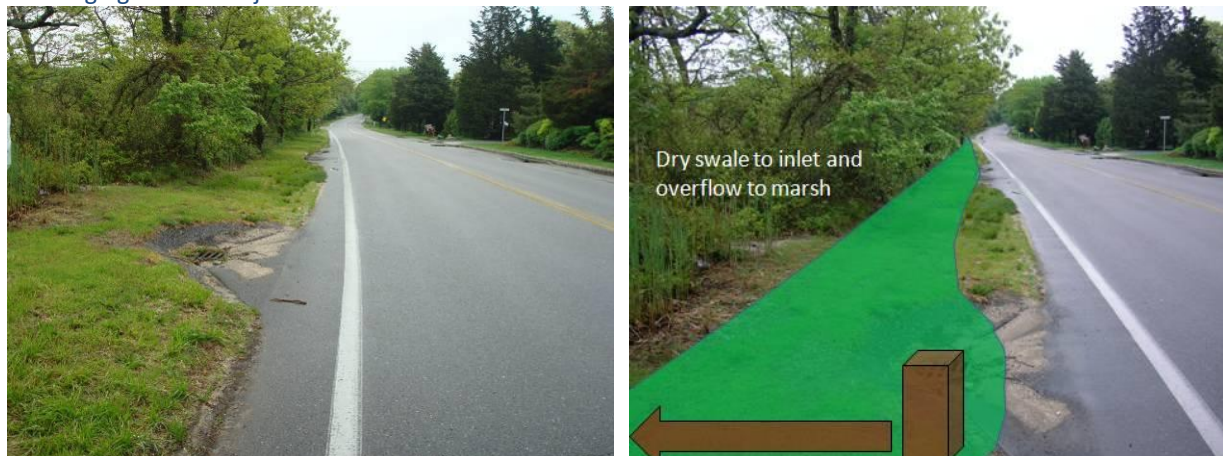
Figure 4.12. Proposed dry swale along Main Bayview Road will allow for improved water quality of stormwater discharging into the adjacent salt marsh.
