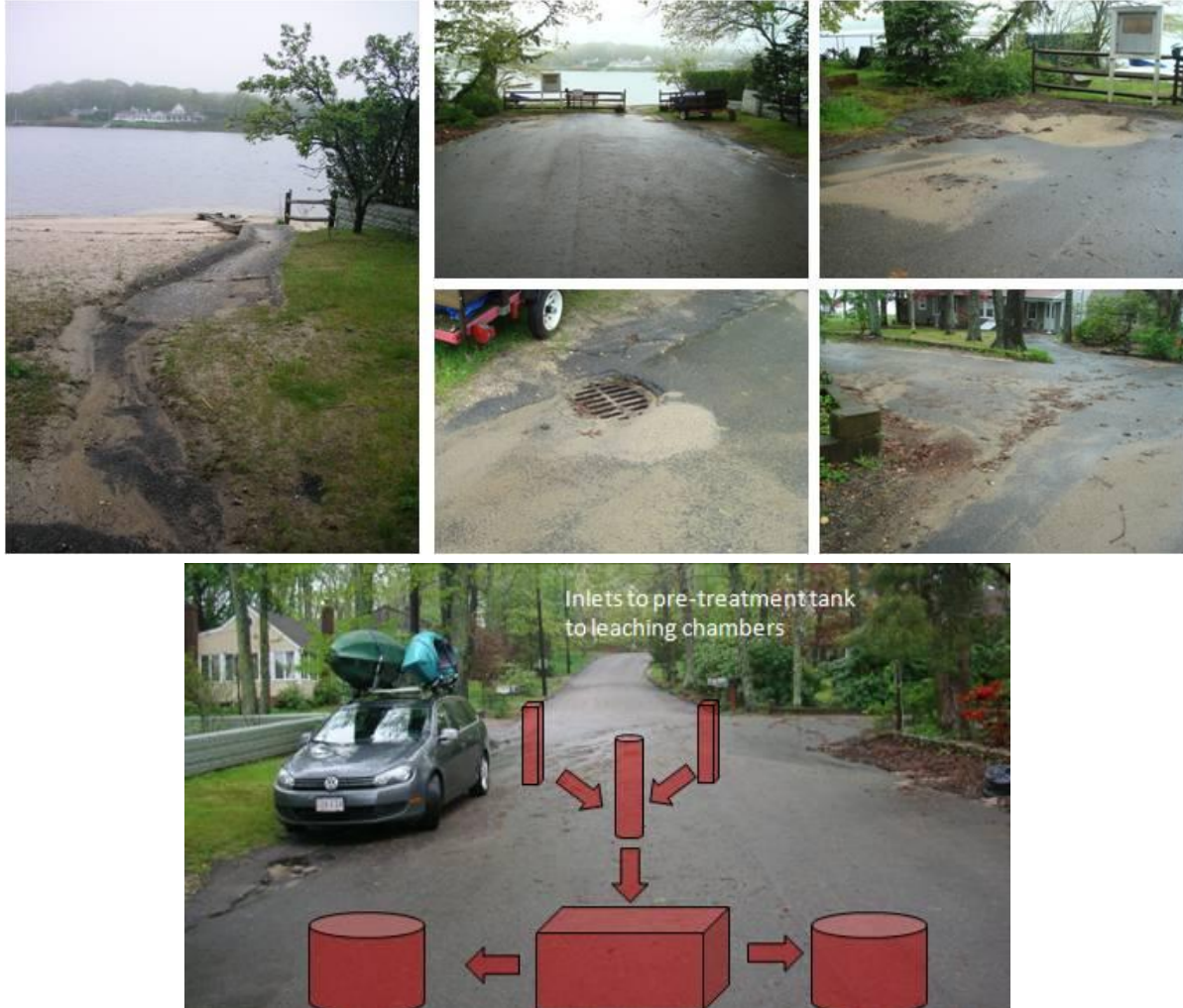
Figure 4.15. Existing conditions along Cedar Avenue where extensive sedimentation has resulted in direct discharge of stormwater into Goose Creek during higher intensity storms (top photos). Proposed retrofit concept would involve more traditional structural measures to accommodate the steep slopes and relatively narrow right-of-way along Cedar Avenue (bottom).
