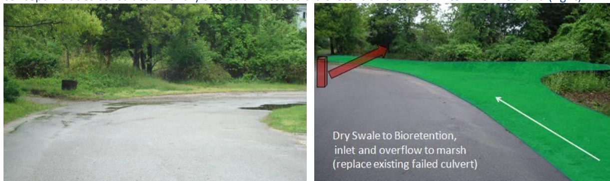
Figure 4.14. Ponding and sedimentation observed at bend in Waterview Drive (left). Proposed stormwater retrofit concept includes construction of dry swales directed to a bioretention area within town-owned land (right).
