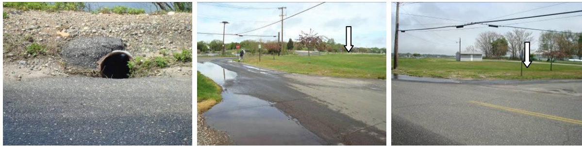
Figure 4.18. Existing conditions along North Bayview Road at the mouth of Goose Creek (top photos). An existing depression within the nearby public park presents an opportunity to repurpose the depression as a bioretention area to improve storage, groundwater recharge, and water quality within the subwatershed (right).
