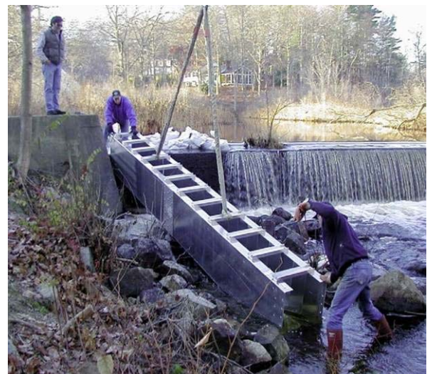
Figure 9: Installation of an Alaska Steeppass structure
