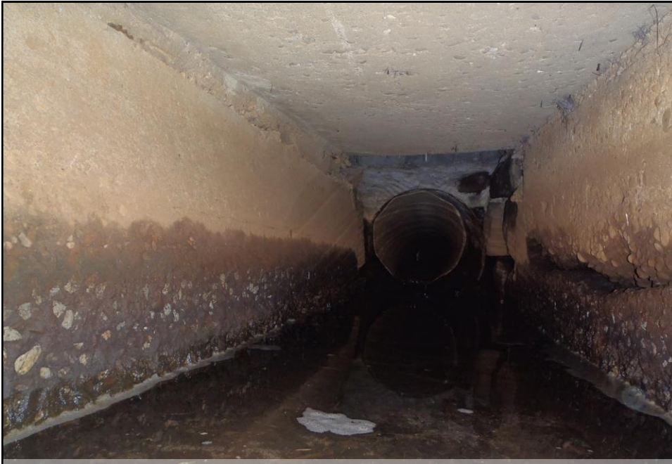
The culvert under Brick Kiln. Note the concrete box transitions to a sliplined corrugated metal pipe with a lip. Not a barrier – but a significant challenge, particularly at low tide
