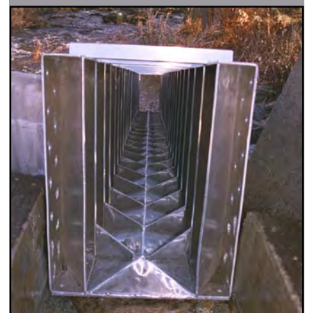
Cross-section: Alaska Steeppass Ladder
