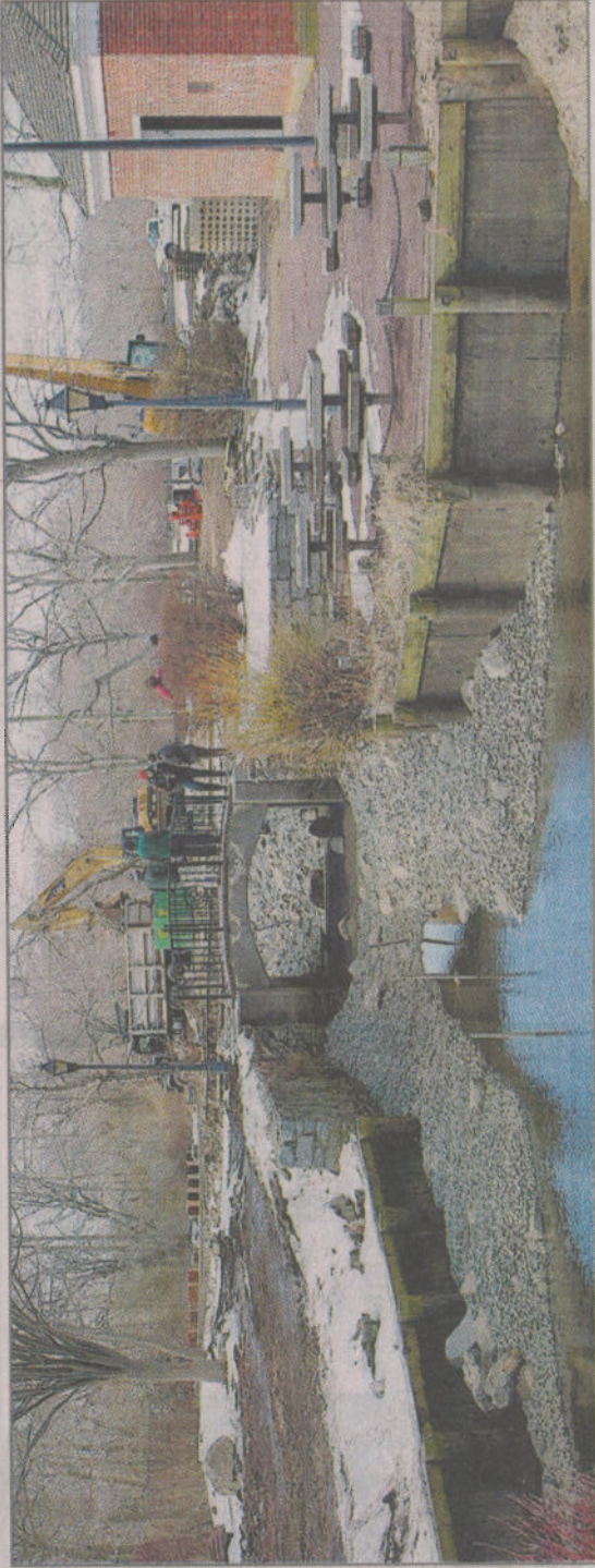
In Riverhead's Grangebel Park a rock ramp has been installed to help alewives scale a dam to spawn upstream in the Peconic River. Alewives are an important food for ospreys, herons, bass and pickerel.
